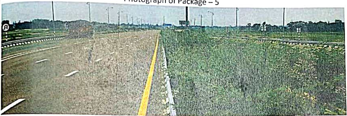
Median Plants at Ch. 183+000
